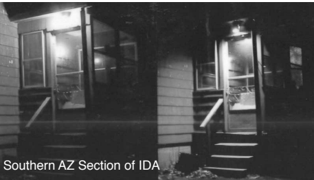
Southern AZ Section of IDA By shielding the light (right side), the bulb was reduced from 60 watts to 40 watts, a 33% savings.
