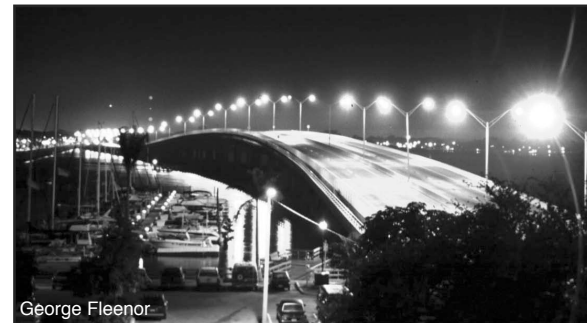
Lighting using drop down glass or plastic lenses can cause unsafe glare.
